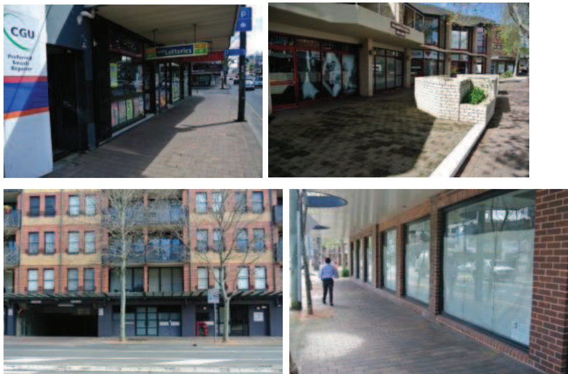
FIGURE 23. EXISTING PUBLIC REALM
